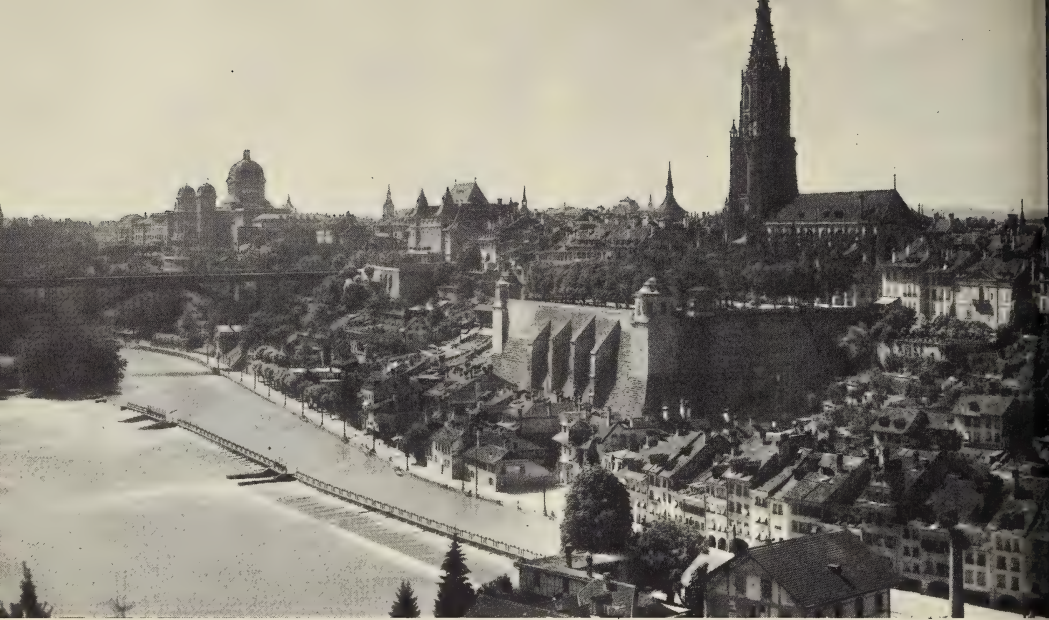
Photograph by Wehrli
